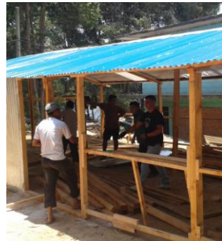
Rebuilding Nagarkot School.
