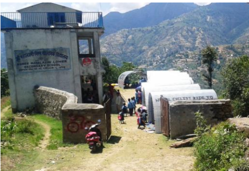
Temporary classrooms at Mahakali School.
